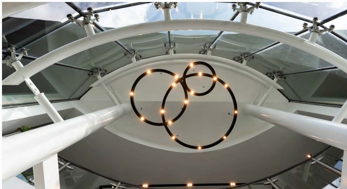
ABOVE | FEATURE LIGHT FITTING
