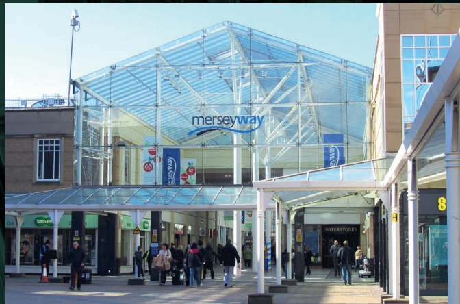
MERSEYWAY SHOPPING CENTRE
